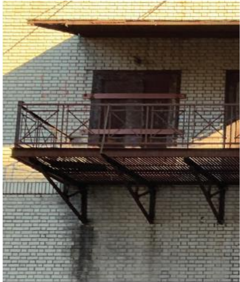
EXISTING THEATER CATWALK
